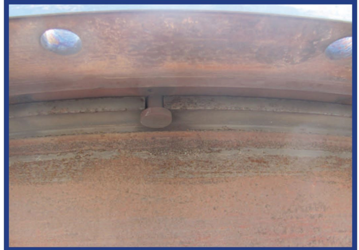
Figure 4: Expansion Pin During Routine Inspection
