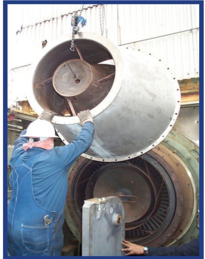
Figure 1: Inlet Annulus Being Installed in the Field
