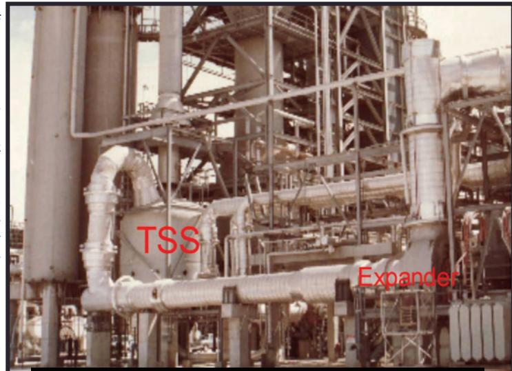
Figure #4—Typical TSS - PRT Installation
