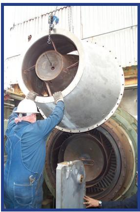
In 1998, RMS was contracted by a major US natural gas company to correct a chronic cracking problem on their Dresser-Clark DJ125 power turbine inlet ducts. The component, called an Inlet Annulus, directs flow from a GE LM1500 gas generator into the DJ125 aero derivative power turbine. Our customer experienced cracking at the Annulus mounting flange which required weld repair on a yearly basis.
