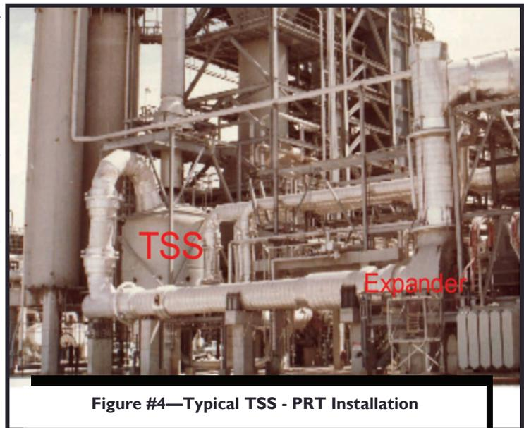
Figure #4—Typical TSS - PRT Installation
